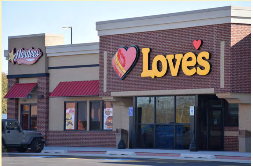
The newly constructed Love's Travel Stop is located in an area where TIF benefits are available for business development and growth. Love's was constructed on land that once was home to Gibson Chevrolet, 1533 East 162nd Street.
